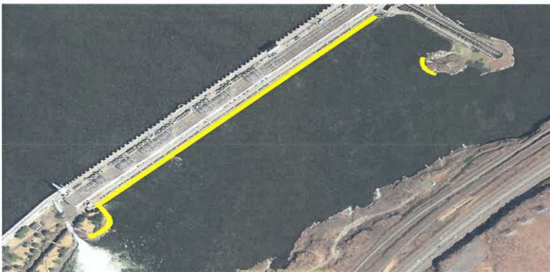
Figure 2. Angling Locations for the 2018 Dam Angling Crew at The Dalles Dam
